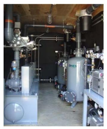
NES was selected to fabricate an SVE/Air Sparge system for a retail petroleum service station in New Jersey. The system was designed and fabricated with dual SVE blowers and dual Sparge compressors to target a vast array of wells along with providing overall redundancy to ensure system operation up-time. Local building codes required that the wooden shed be designed and constructed in accordance with the International Building Code (IBC).
